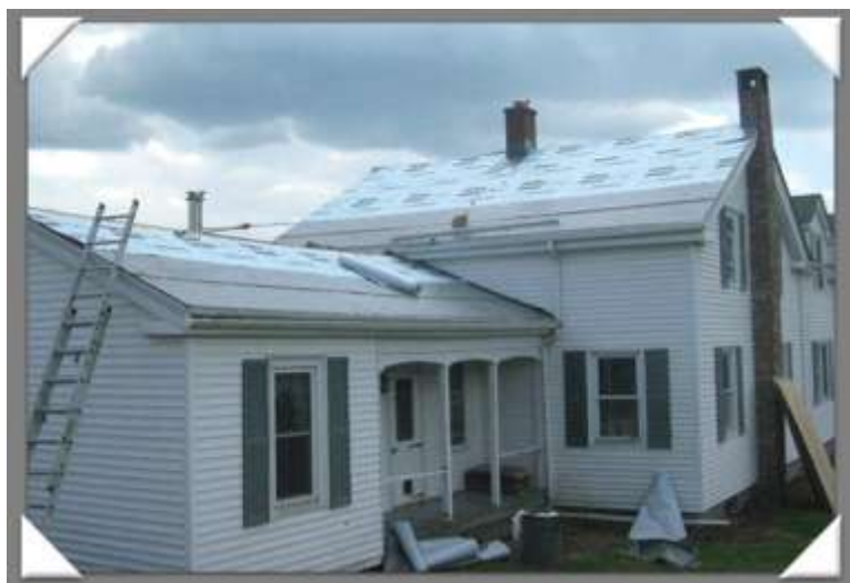
Installation of New Roof on PPAS Farm House
