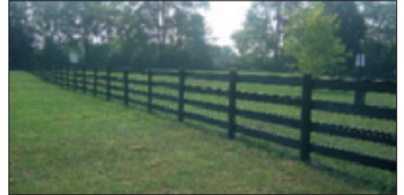
Completed 4-board perimeter fencing.
